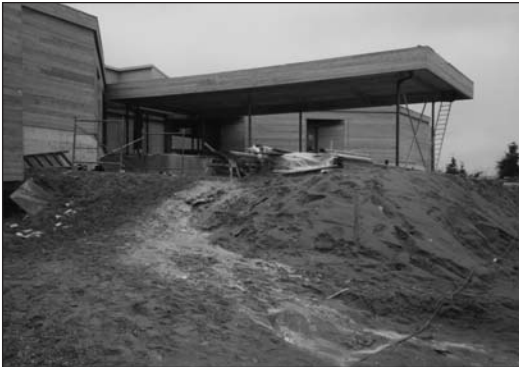
Club entry under construction.
