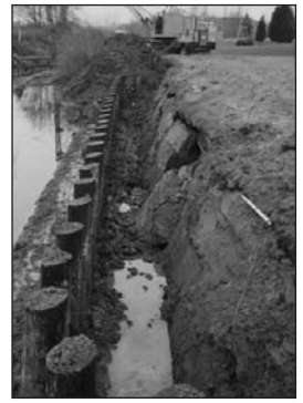
Construction of Richmond/ Gleneagles dikes.
