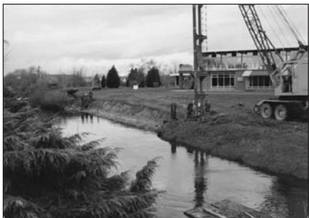
Construction on Richmond/Gleneagles golf course, March 1959.
